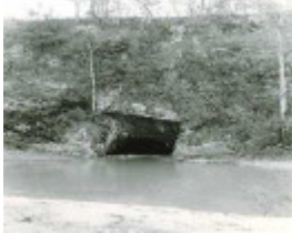
B3121 Pound Bend Tunnel
