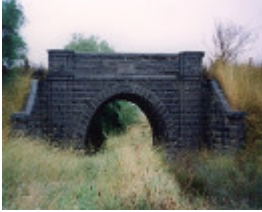
B1180 Corkscrew Bridge, Calder Hwy, Diggers Rest
