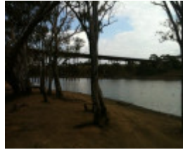
B3741 Melton Viaduct Railway Bridge
