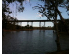
B3741 Melton Viaduct Railway Bridge
