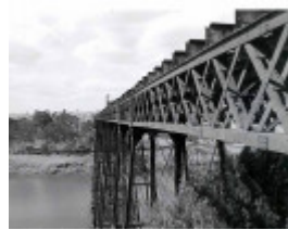
B3741 Railway Viaduct Melton
