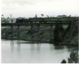
B3741 Viaduct Railway Bridge
