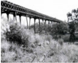
B3741 Railway Viaduct Melton
