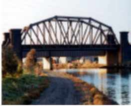
B5745 Rail Bridge over Maribyrnong River
