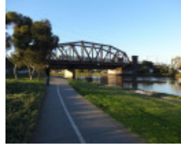
B5745 Rail Bridge over Maribyrnong River
