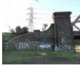
B5745 Rail Bridge over Maribyrnong River abutment
