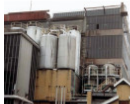
B5089 Main Refinery & New Boiler
