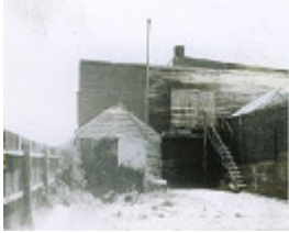
B4197 Old Bakery Building
