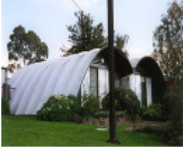
B4835 Former Supermarket
