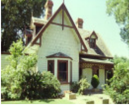
B6573 Swiss Cottage - Former Curator's Lodge
