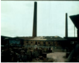
B5546 Frmr Hoffman Brickworks
