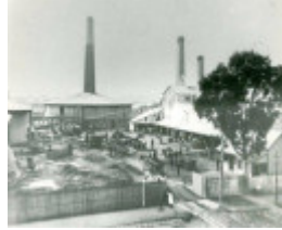
B5546 Frmr Hoffman Brickworks
