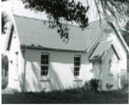
B1724 Progress Hall Flinders Rd Shoreham
