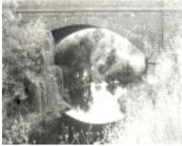
B0941 Bluestone Bridge
