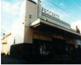
B7008 Progress Hall
