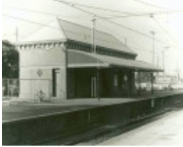
B4933 Moreland Rail Station
