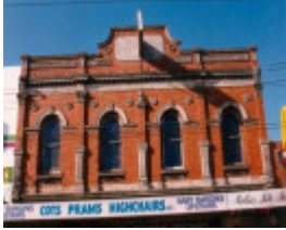
B6707 First Floor Facade H.Bates Building
