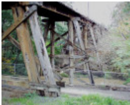
B4173 Eltham Rail Bridge
