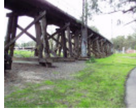
B4173 Eltham Rail Bridge
