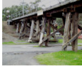
B4173 Eltham Rail Bridge
