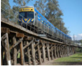
B4173 Eltham Rail Bridge
