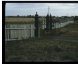
SEXTON'S COTTAGE SITE, SOUTH PORTLAND CEMETERY
