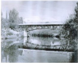
B7215 Macrobertson Bridge
