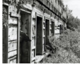
B2165 Former Living Quarters now Stores
