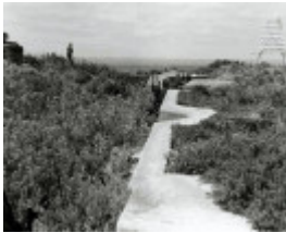
B2165 South Channel Fort Fire Control on Left
