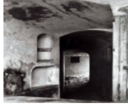
B2165 Corridor Linking Gunposts with Observation Points
