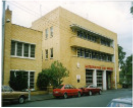
B6651 Fire station & Flats
