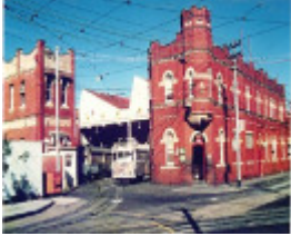
B6152 Malvern Tram Depot
