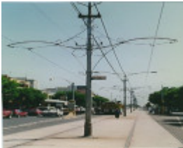
B6438 Ornamental Tram Poles
