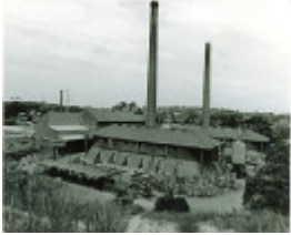
B4534 Menzies Park Brickworks
