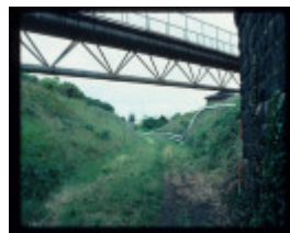
RAILWAY BRIDGE AND CUTTING
