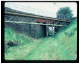
RAILWAY BRIDGE AND CUTTING
