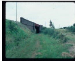
RAILWAY BRIDGE AND CUTTING
