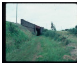
RAILWAY BRIDGE AND CUTTING
