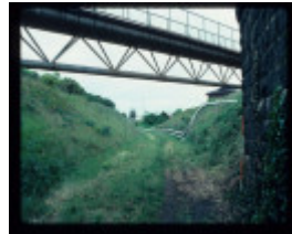
RAILWAY BRIDGE AND CUTTING
