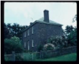
WATTLE HILL HOUSE, WILSONS RD, PORTLAND WEST
