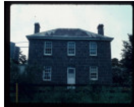
WATTLE HILL HOUSE, WILSONS RD, PORTLAND WEST
