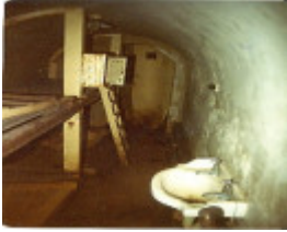
B5603 Air Raid Shelter
