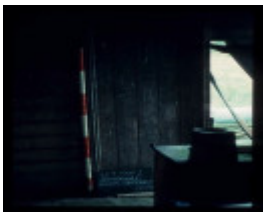
LAKE CONDAH - COMPLEX D (MURPHY'S HUT) FEATURE - INTERNAL DOOR KITCHEN
