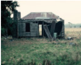
6675 33 Feature 1 South wall of hut
