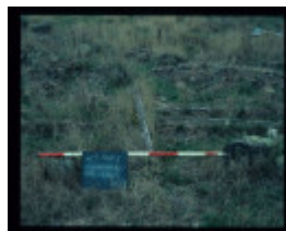
LAKE CONDAH - COMPLEX D (MURPHY'S HUT) FEATURE - COLLAPSED POST RAIL FENCE
