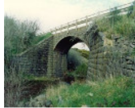
B6074 Bridge Inn Road Bridge
