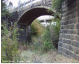
B6074 Bridge Inn Road Bridge
