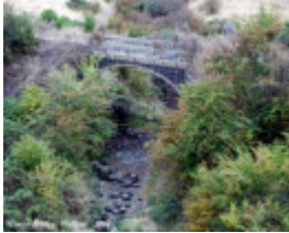
B6074 Bridge Inn Road Bridge
