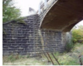
B6074 Bridge Inn Road Bridge
