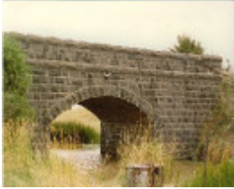
B1577 Bluestone Bridge
