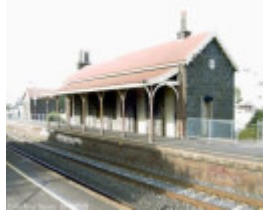
B2285 Rail Station
