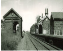
B2285 Railway Station & Goods Shed
