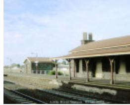
B2285 Rail Station
