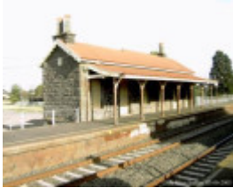
B2285 Rail Station
