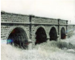
B2055 Rothwell Bridge
