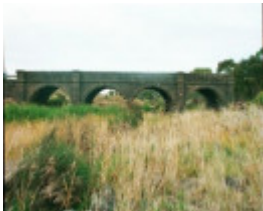
B2055 Rothwell Bridge
