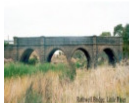
B2055 Rothwell Bridge
