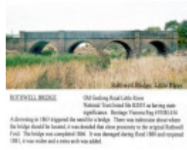
B2055 Rothwell Bridge
