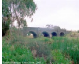
B2055 Rothwell Bridge
