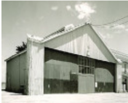
B4310 Building No 104
