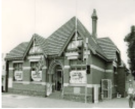
B5072 Former Shire Hall
