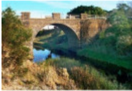
B2782 Grant's Bridge
