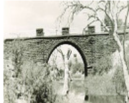
B2782 Grant's Bridge
