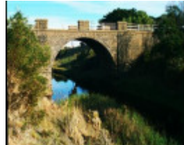
B2782 Grant's Bridge
