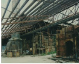
B6492 Wunderlich Terra Cotta Roof Tile Works
