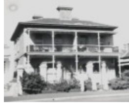
B3414 19-21 Alfred Crescent Fitzroy North
