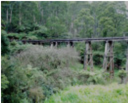
B2960 Puffing Billy Trestle Bridge
