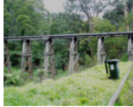
B2960 Puffing Billy Trestle Bridge
