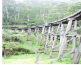
B2960 Puffing Billy Trestle Bridge
