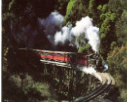
B2960 Puffing Billy Trestle Bridge
