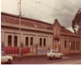
B4138 Fmr Cable Tram Depot
