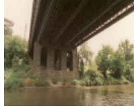
B6649 Hawthorn Bridge
