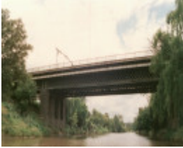
B6649 Hawthorn Bridge
