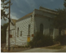
B5448 Former Mechanics Institute
