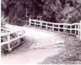
B7032 Myrtle Creek Bridge
