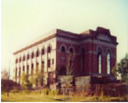
B5903 Former Substation
