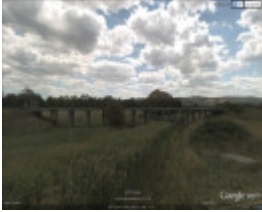
B7069 Stringybark Creek Bridge
