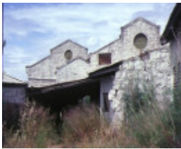
former melbourne meat preserving company buildings van ness ave maidstone side elevation dec1981
