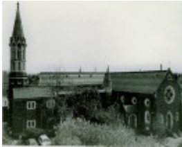
B3718 St Joseph's Building
