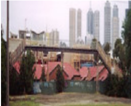
B7125 Nth Fitzroy Railway Footbridge
