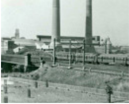
B6586 Fmr Richmond Power Station
