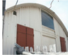
67162 B5311 Iron Store SW facade
