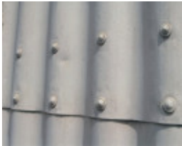
67162 B5311 Iron Store detail NW facade
