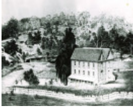
B3139 Dight's Water Mill
