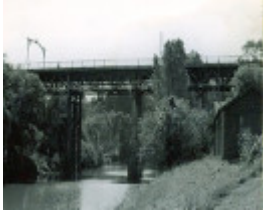
B1599 Victoria St Bridge
