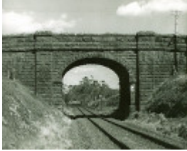
B3166 Navigators Railway Bridge
